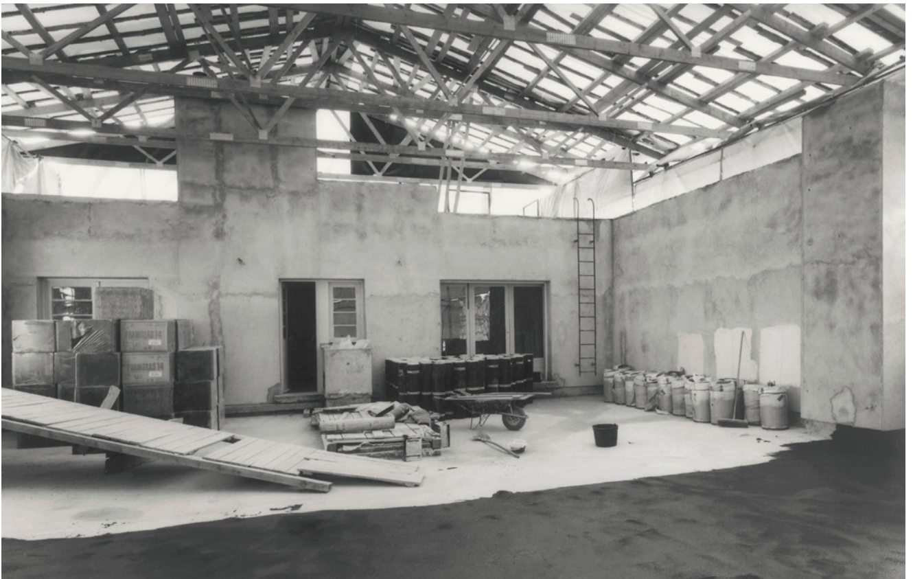
Fig. 10: Condition of the terrace prior to reconstruction, 1998
